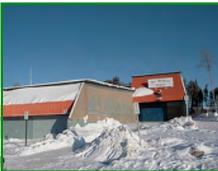
The Uniplex (Evacuation Centre)
