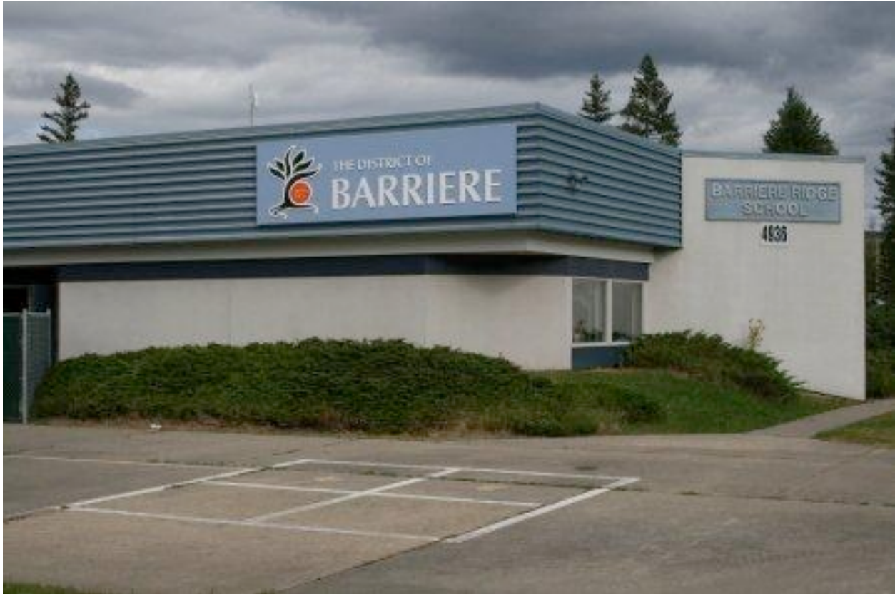
Photo courtesy of the District of Barriere
